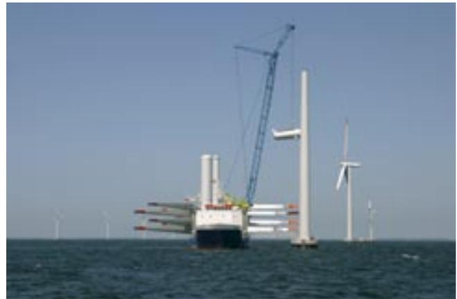
submarine, and Van Oord ACZ, an offshore sector construction and installation contractor. Other shareholders are Hovago Cranes (part of the Baris Group) and Marine Construct. The new company operates the purpose-built Jumping Jack (shown in Figure 5.8), a jack-up barge with an onboard crane, which was used to install the Horns Rev foundations.
